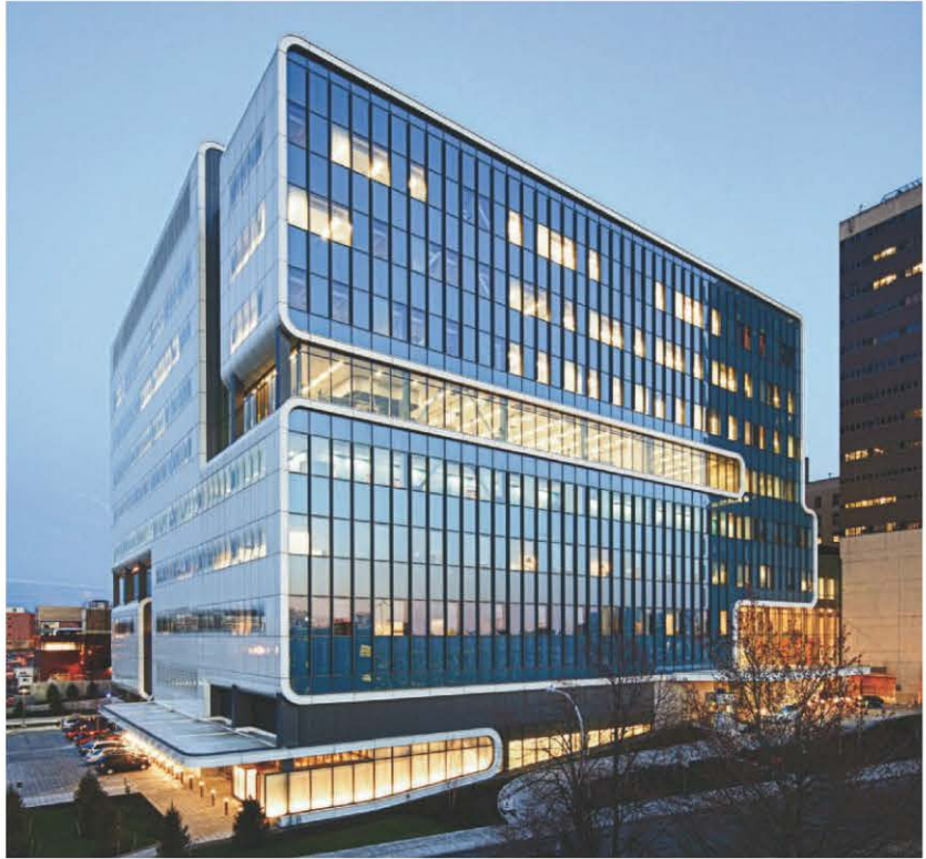
MIND MELD The building’s 476,000 square feet integrates a vertical core and a horizontal structure that embody the clients’ cooperative philosophy of sharing knowledge. The facade combines complementary yet contrasting zones of enameled panels and curtain walls, laced together by a sinuous metal ribbon.
